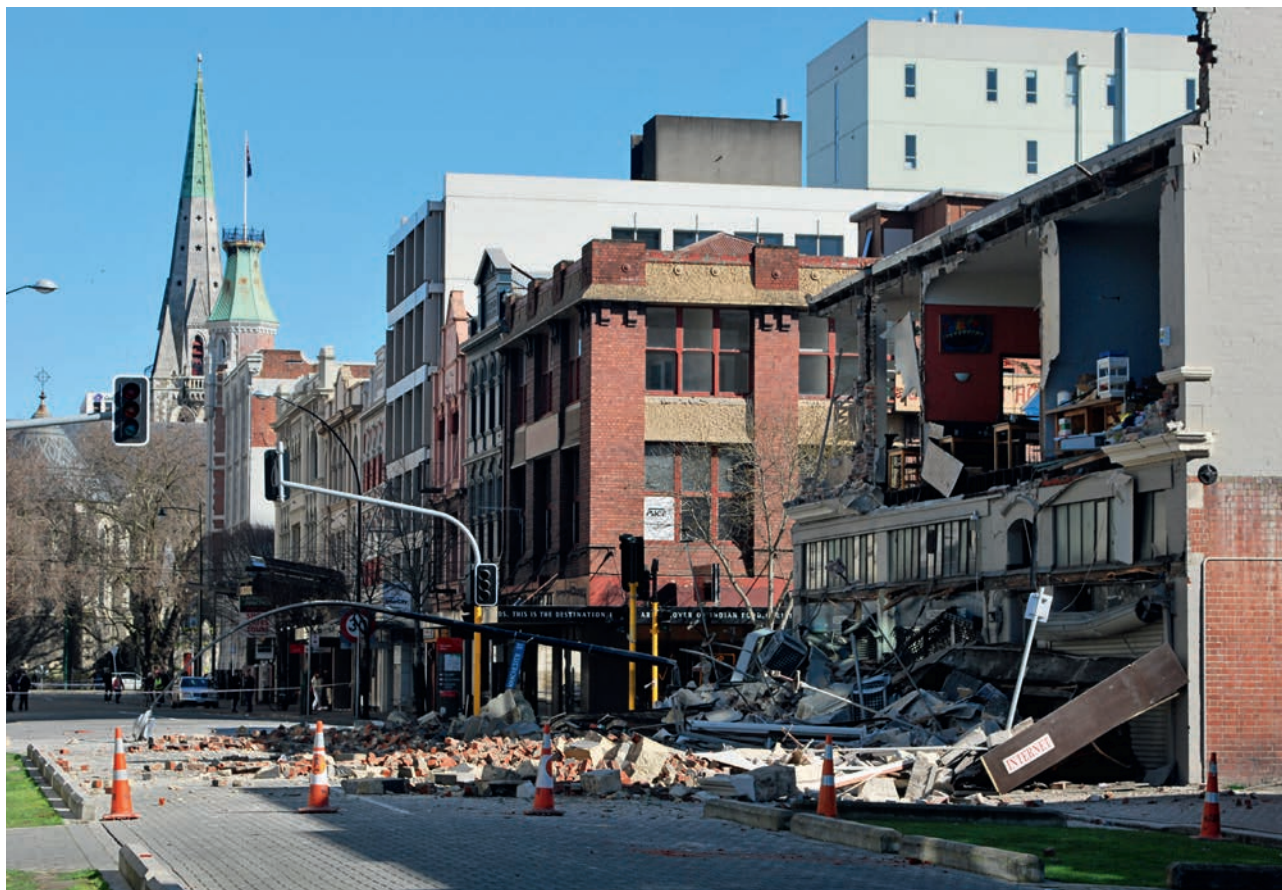
Above: The damage in New Zealand's Christchurch caused by the 22 February 2011 earthquake
