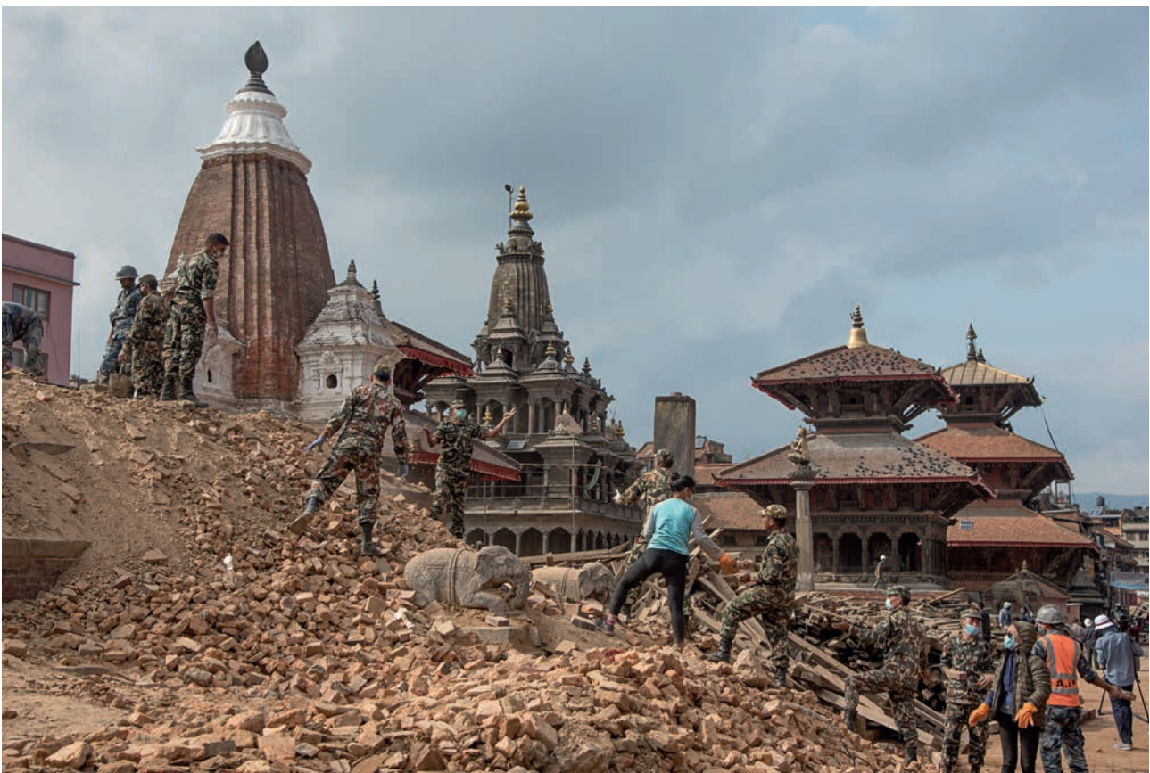
Above: The destruction in Patan Darbar Square in Kathmandu, Nepal, after the major earthquake on 25 April 2015
