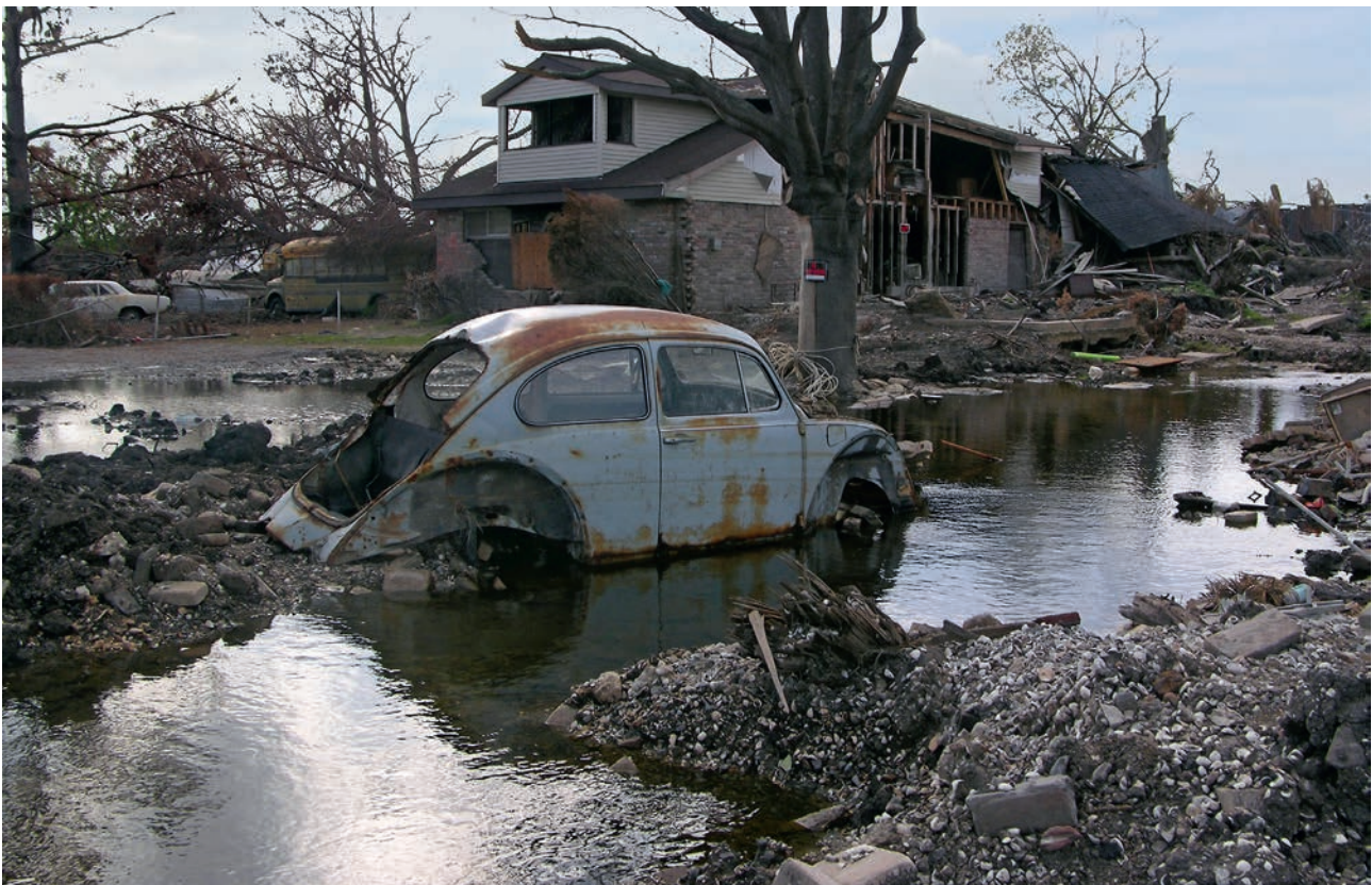
Above: Water leakage from the New Orleans levee three months after Hurricane Katrina hit on 23 August 2005
